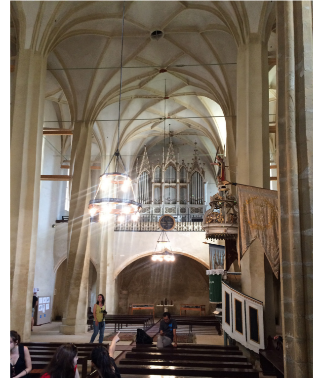
the structural reinforcement in the main hall
